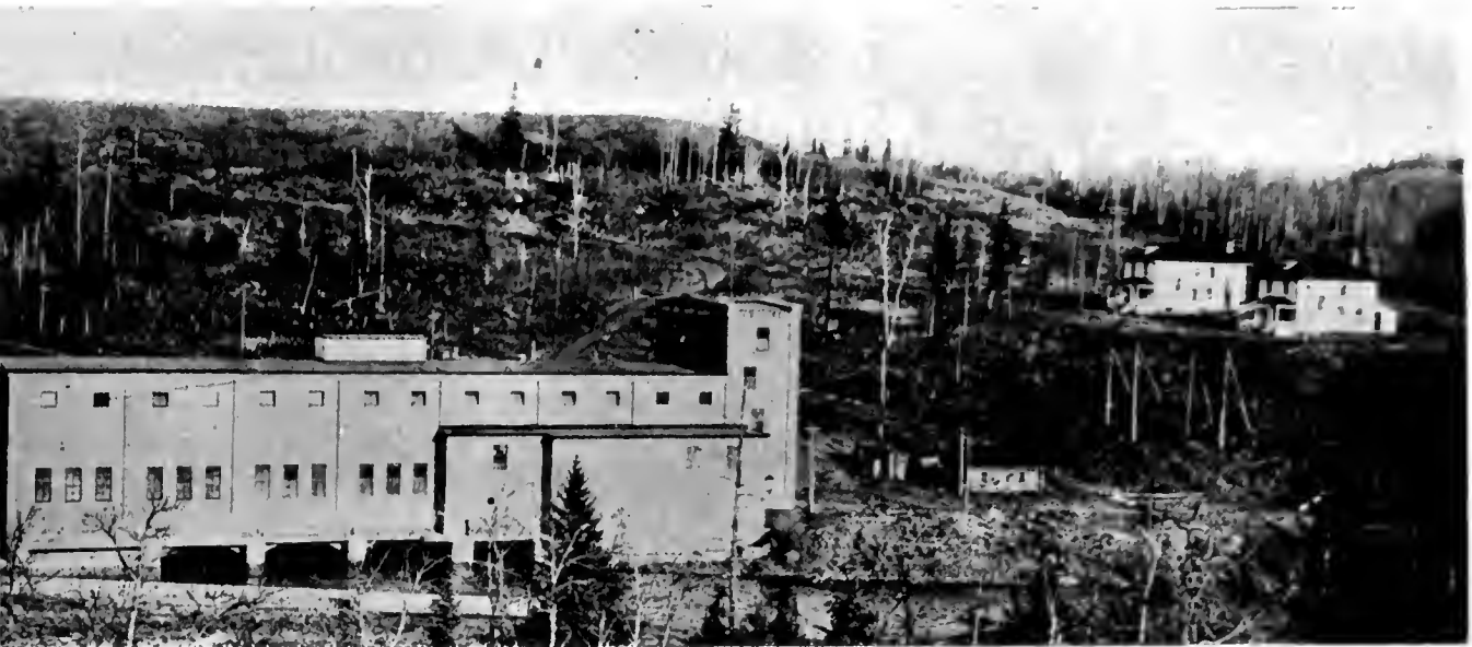
Reinforced Concrete Power House and Tall Race—Kaminlstiqua River In Foreground and Transmission Line to the Right.
